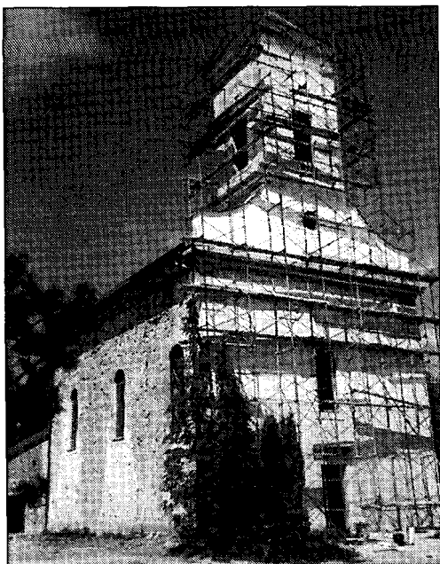
Church of St. Rok, under restoration, 1998.
