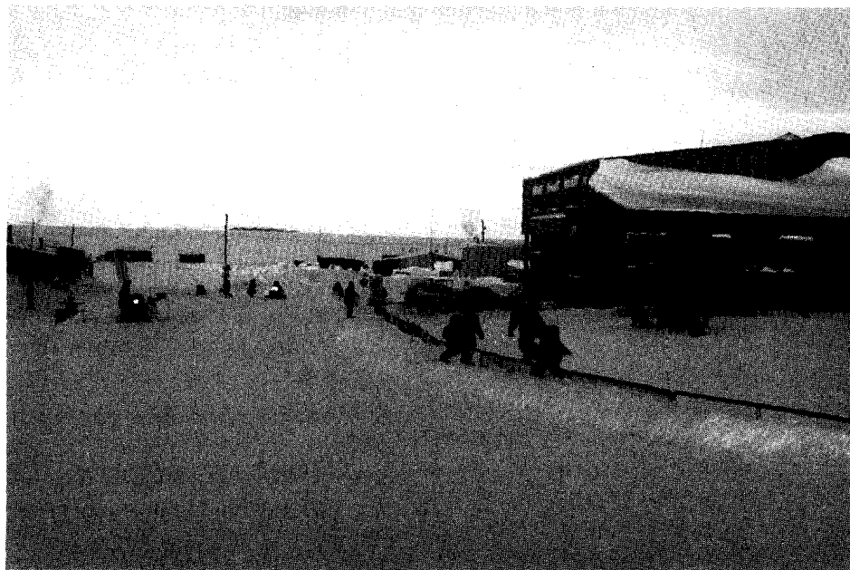
The Jimmy Hikok Elementary School in Kugluktuk was built with funds from the "Impact and Benefits Agreement" that BHP Billiton negotiated with the Kitikmeot Inuit Association. Photo: Patricia Simpson
