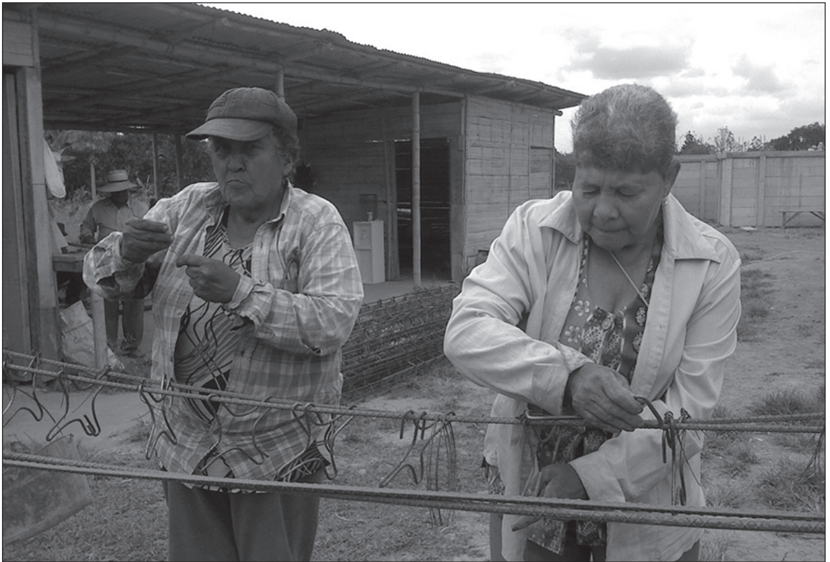
Nashira under construction.
