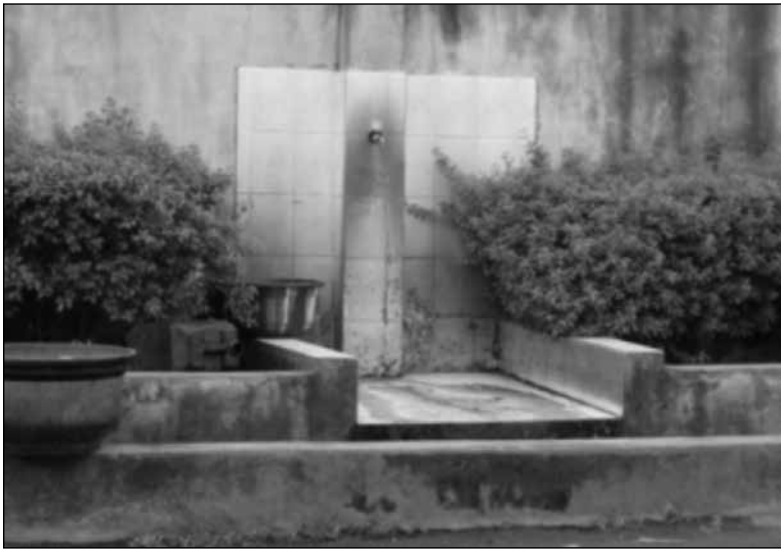
Photo 5: Borehole water point outside a house. Source: authors' fieldwork.
